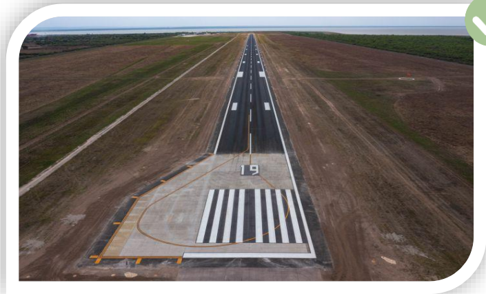
Rio Hondo Runway and new lighting system (September 2023)
